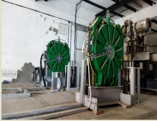
Energy efficient gearless elevators Disconnection of 2x80 KVA & 2X20 kVa UPS
